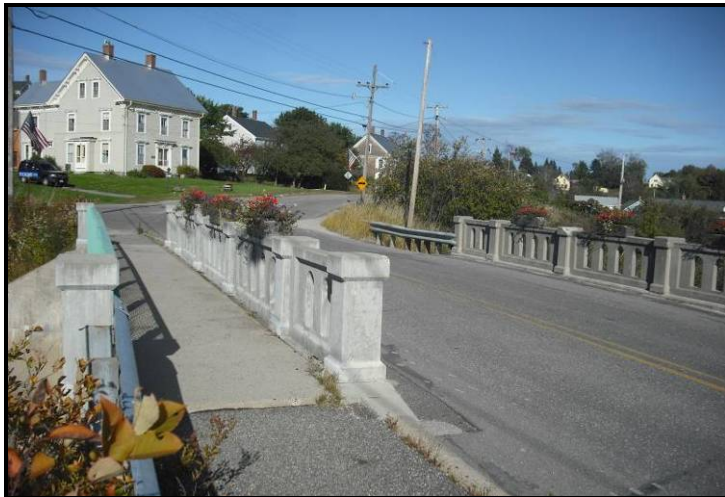
Planter boxes on line the pedestrian crossing structure on the bridge across the Pleasant River in Columbia Falls. Photo: WCCOG
