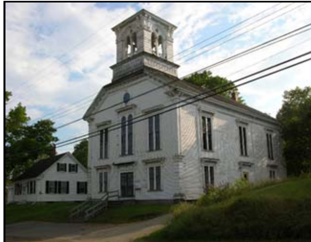
Renovations are underway way to restore Liberty Hall, One of four structures in Machiasport listed on the National Register of Historic Places.
